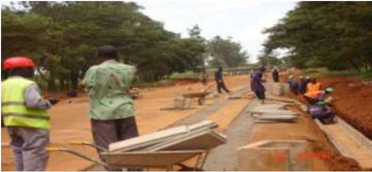
Company, Drainage Works
